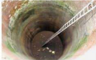
Figure 1: Excavated Ajnala well
